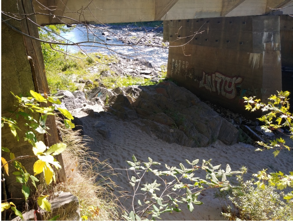
Photo: Visible outcropping bedrock between Pier 3 and North Abutment: (note near vertical dip and variation in elevation)
